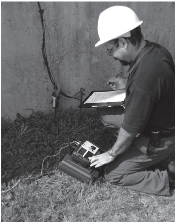
Using ART method with Megger DET3 Series to test commercial earth (ground) without disconnecting the system
